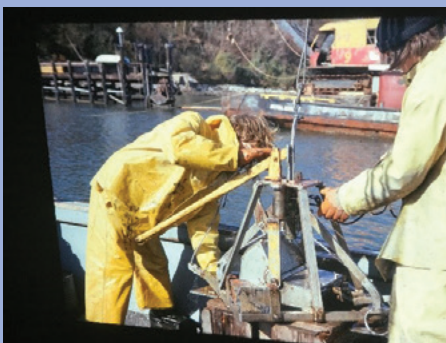
Smith-McIntyre benthic grab used for sampling benthic communities of Narragansett Bay in early 1970s
